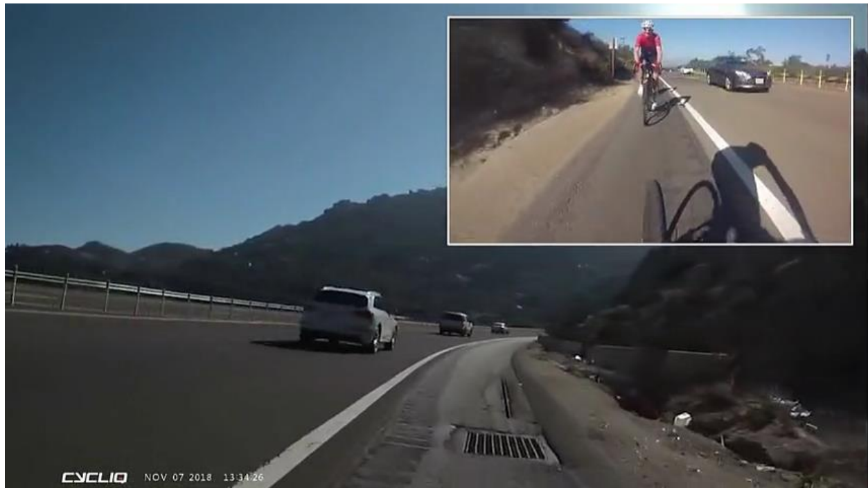
Figure 1. Grate squeeze right of rumble strips southbound, narrow shoulder, just before Ramona Summit.
