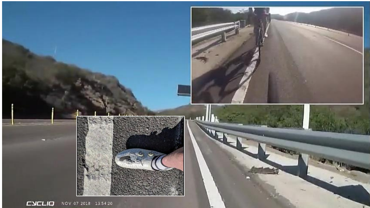
Figure 5. Uphill northbound, half way between Scripps Poway Parkway and Poway Rd, super narrow rumble strip trap at guardrail.
