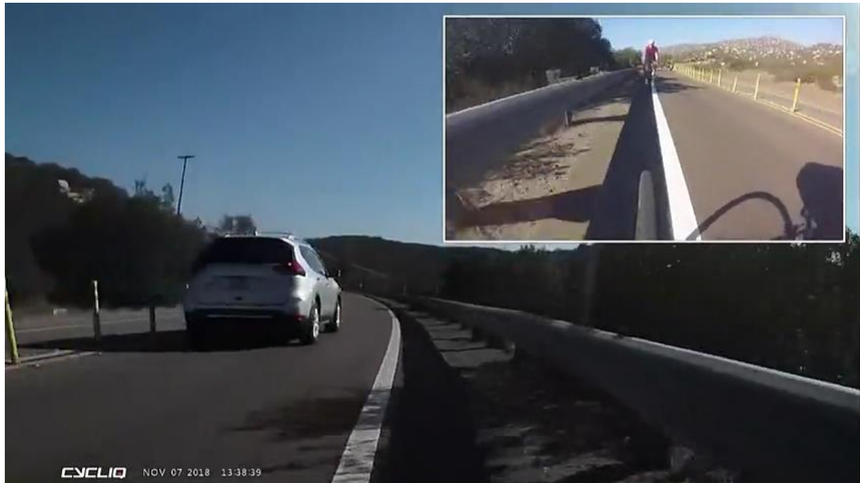
Figure 2. Downhill southbound 1 lane, rumble strips, squeeze at guardrail, super narrow shoulder, centerline delineators, EXTREMELY DANGEROUS.
