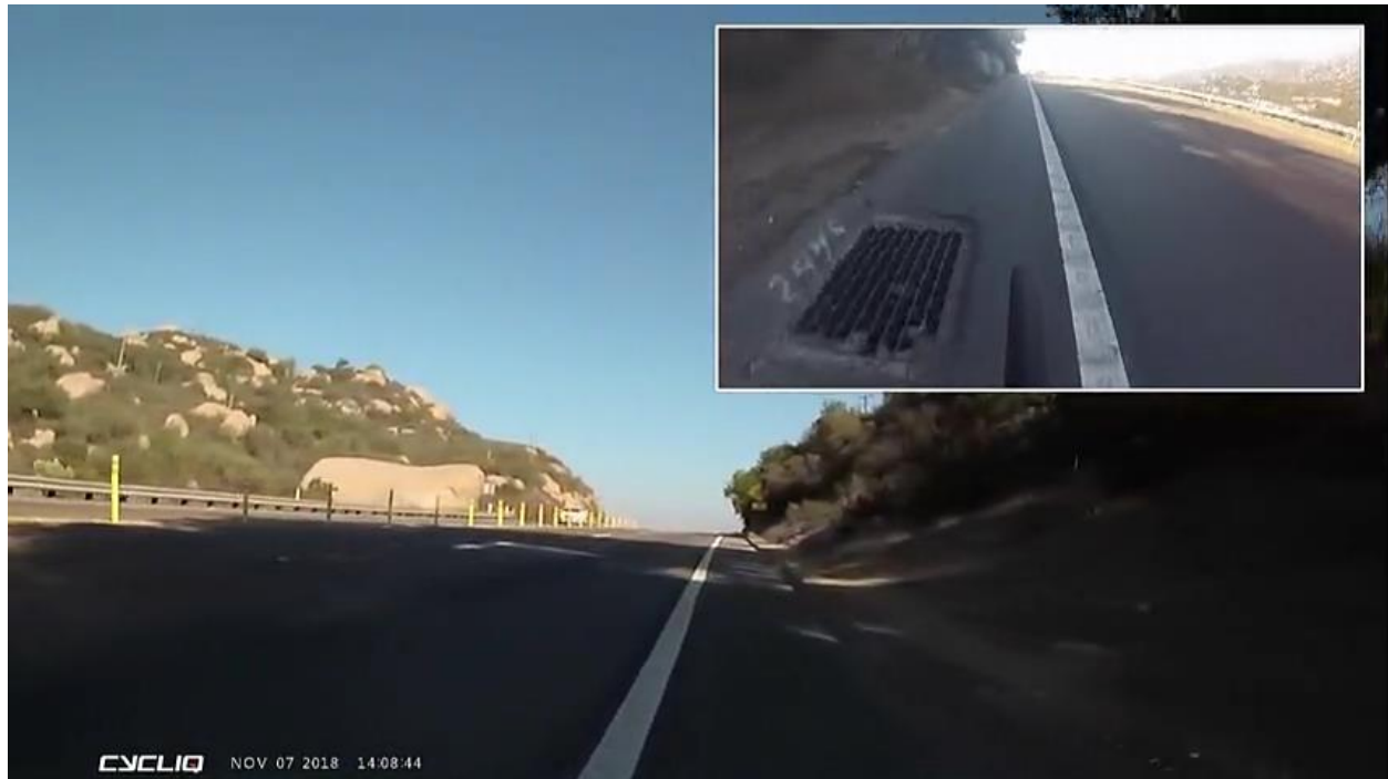
Figure 9. Approaching Ramona Summit northbound, 2 lanes, rumble strips, narrow shoulder with drains and debris.
