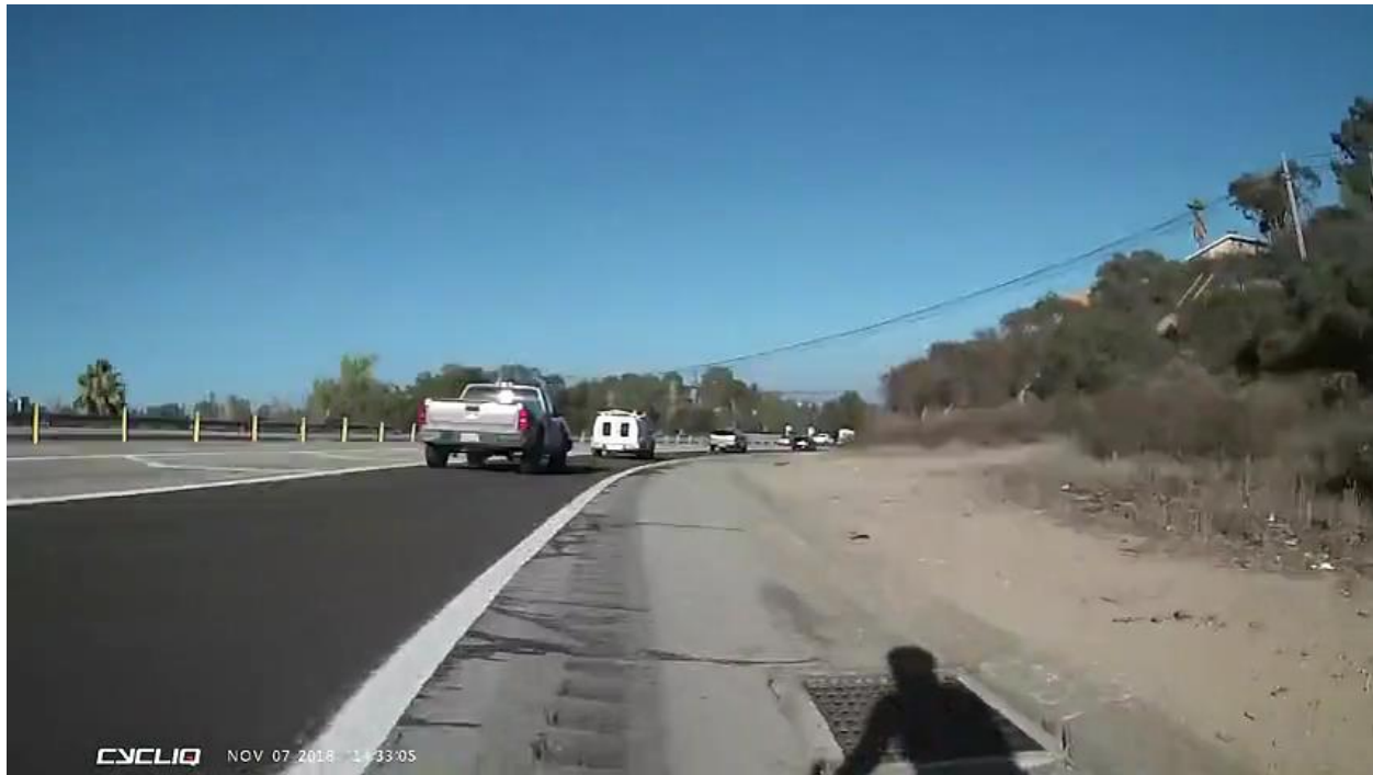
Figure 10. Approaching Archie Moore northbound, rumble strips trap left turning cyclists.
